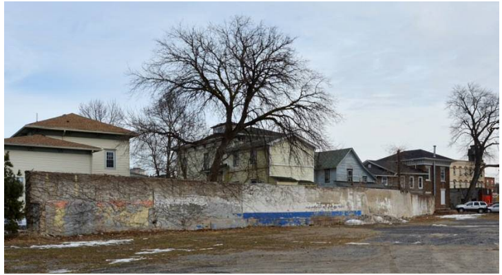
The wall at 131 Water Street in 2014
